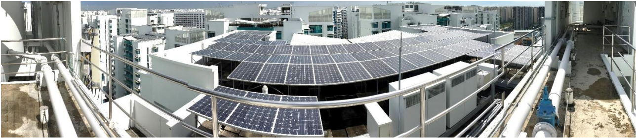
Figure 1: Panoramic view of the PV panels installed on the rooftop of Blk183 of the Edgefield Plains precinct, Punggol new town, Singapore. (Source: the authors)
