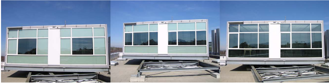
Fig. 1. Photographs of the Fraunhofer ISE test facility with the three window configurations (left: small window, middle: medium window, right: large window). The rooms can be rotated fully in order to be more or less independent on seasons to set up a defined angle of incidence for the sun.
